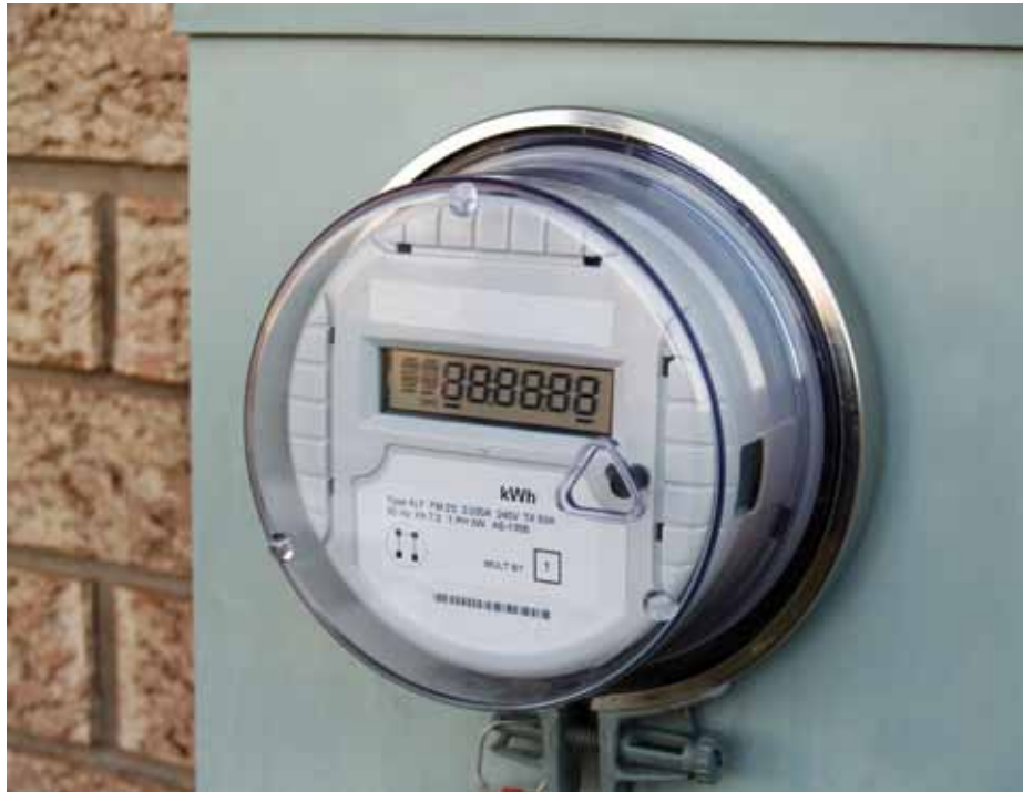
A smart meter provides an even greater level of detail of a customer's actual power use and is known to be the future of meter technology. It can read data in real time and can send data back to the utility company about how and when power is used at a particular site. A smart meter has built-in power-quality monitoring and can also send power-outage notifications back to the utility company. ©iStockphoto.com/Trevor Fisher
